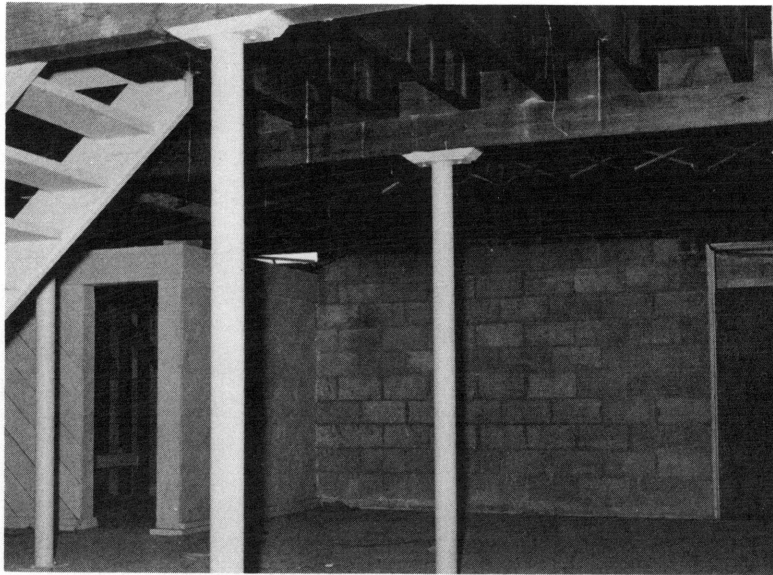
Fig. 2.15—The 2SB house basement.
